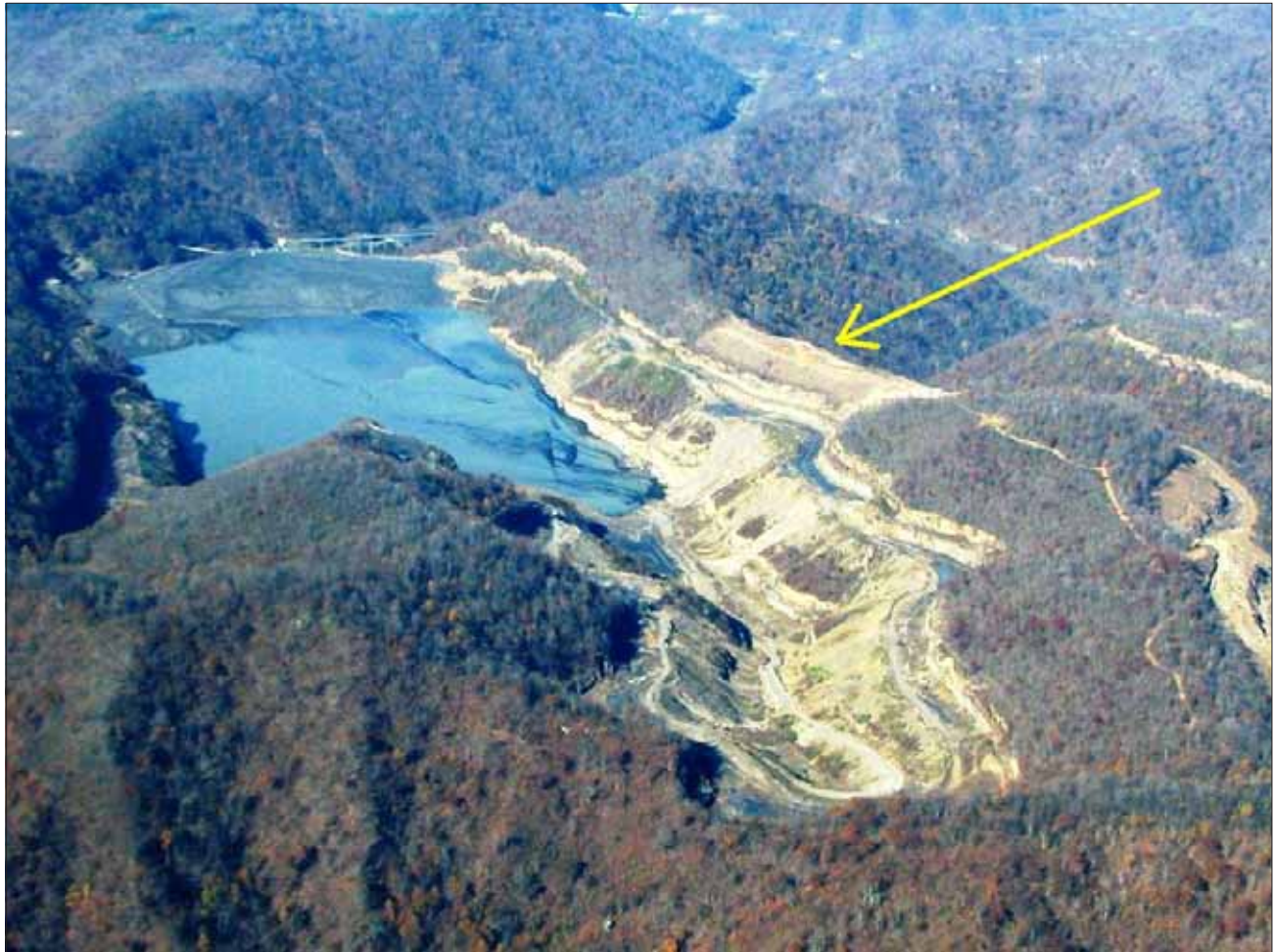
The arrow marks where clearing and blasting have started on Massey's Bee Tree permit on Coal River Mountain. The "lake" to the left of the blasting site is the billions of gallons of toxic goo held back by the Brushy Fork coal slurry dam. Photo by Vivian Stockman. Flyover courtesy SouthWings.
