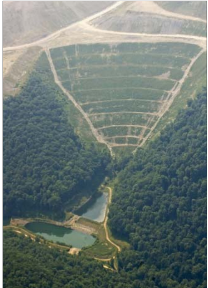
A valley fill with the Corps’ idea of “streams” on either side. Hurry along folks, no significant impacts to be seen here. photo by Giles Ashford, www.ashford7.com. a six-day trial in Huntington in October 2006.
