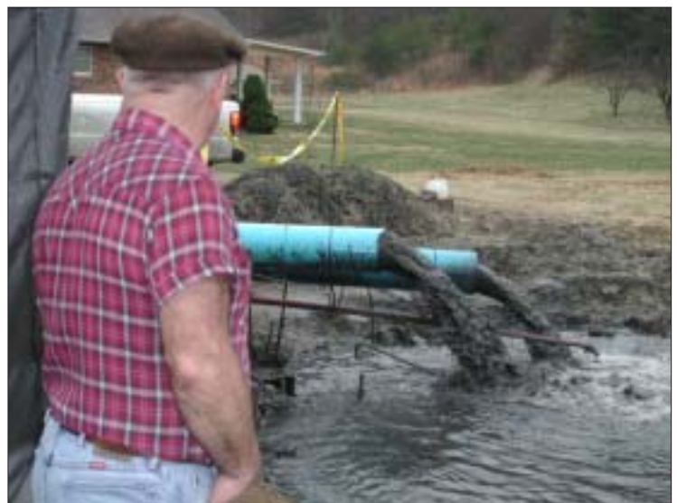
Cleanup continues three months after a huge Massey subsidiary’s coal sludge spill in Martin County, Ky. - the largest environmental disaster in the southeastern US.
