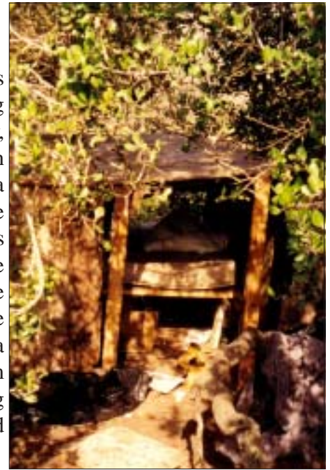
Typical "housing" for migrant farm laborers, adjacent to strawberry fields near San Diego, Calif.
