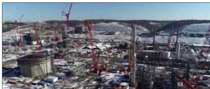
Above: A still from drone footage taken by Nick Hood of the construction of the Shell cracker plant near Pittsburgh, PA. This footage and more shot by OVEC's Alex Cole is part of our YouTube series by Evan Gilland about the proposed Appalachian Storage Hub.
