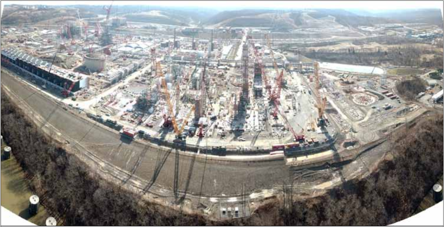
Above: A Shell cracker plant under construction along the Ohio River near Beaver, PA. This huge industrial facility is one of five or more such plants that would be part of the proposed Appalachian Storage Hub.
