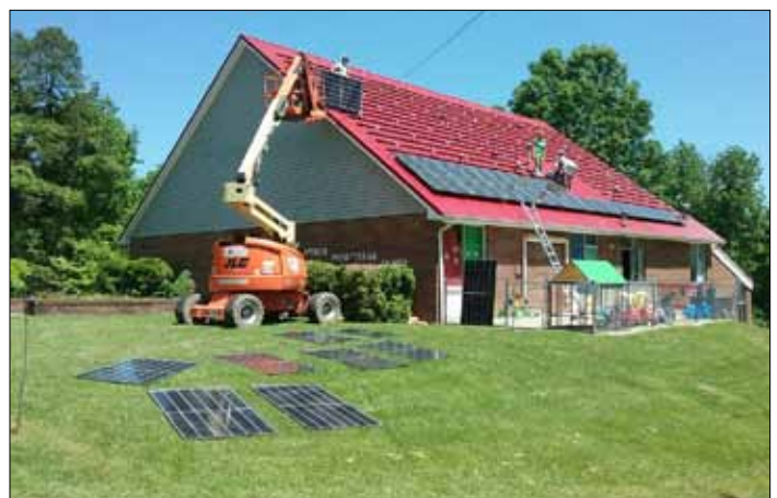
Solar panels going on the church in May. Photo courtesy SPC.
