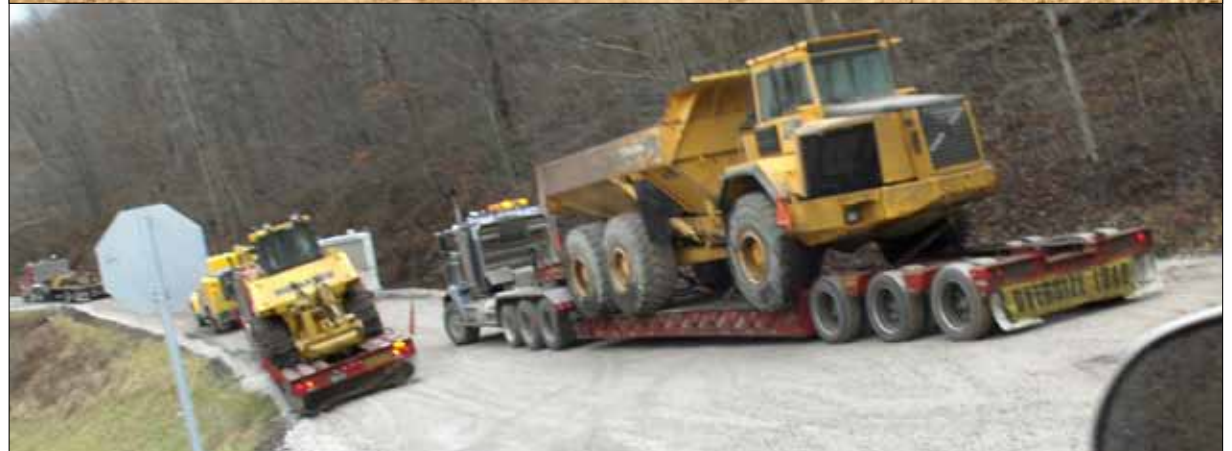
Top-most photo: A well pad under preparation in Wetzel County, WV. Above: The big earth moving equipment used in well pad prep sometimes has trouble making its way to the well pad.
