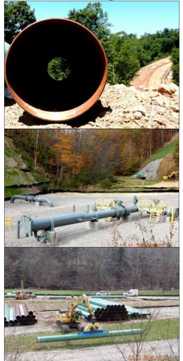
Above: Assorted pipeline-related activity in Wetzel County, WV. The pipeline in the top and bottom photos is 30 inches in diameter. Photos by Bill Hughes.
