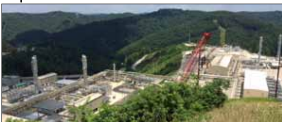
Gas processing plant in Wetzel County, WV.
