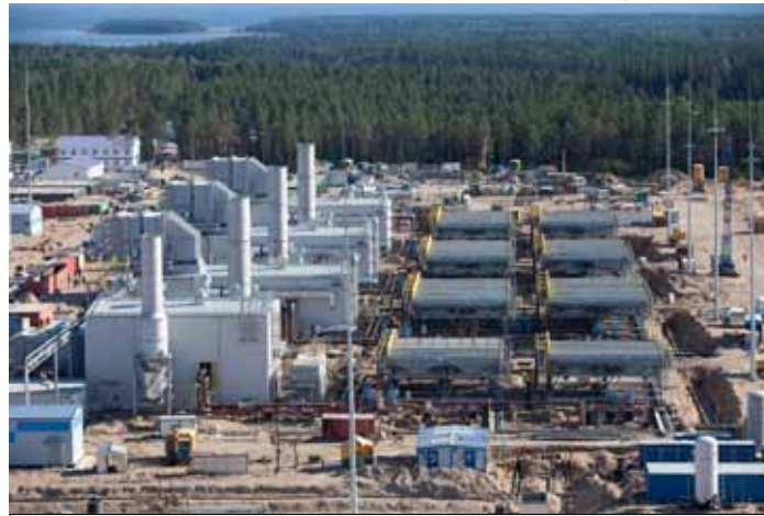
What one compressor station for a 46-inch pipeline looks like. The proposed pipeline would be 42 inches in diameter and 550 miles long, stretching from PA to NC. Photo courtesy WVWL.
