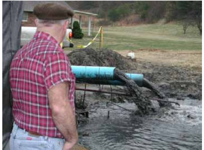
Above: In March, 2001, Inez, KY resident Monroe Cassady looks on at continued clean-up efforts five months after the Martin County coal sludge impoundment disaster.
