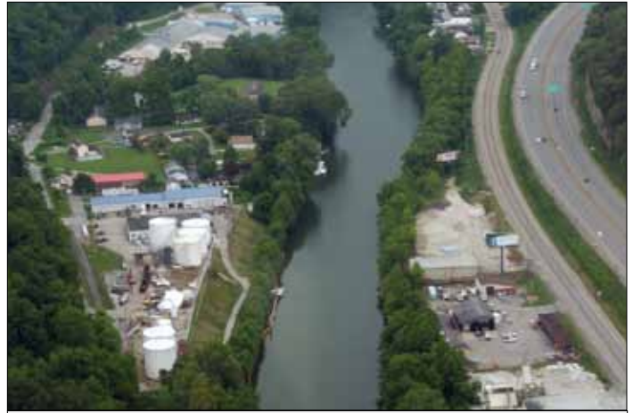
Above: On July 23, demolition was well underway at the Freedom Industries tank farm, seen here in the foreground on the left bank of the Elk River. Just 1.5 miles downriver (toward the top of the photo) is WV American Water's drinking water intake valve. On August 17 the Charleston Gazette reported: "Back in April 2006, officials from West Virginia American Water told state regulators they were planning to review the Elk River watershed to find out what potential contamination sources were upstream from their Kanawha Valley water treatment plant... Three times over a two-year period, West Virginia American officials marked a 'P' — meaning 'Planning to do' — next to a question about whether the company was going to 'review' the treatment plant's watershed 'for potential contaminant sources.' The review was not completed — and it still hasn't been."
