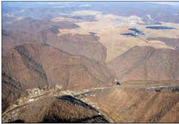
Even when a MTR site is "reclaimed," pollution coming off valley fills does not magically disappear. Flyover courtesy SouthWings.org.
