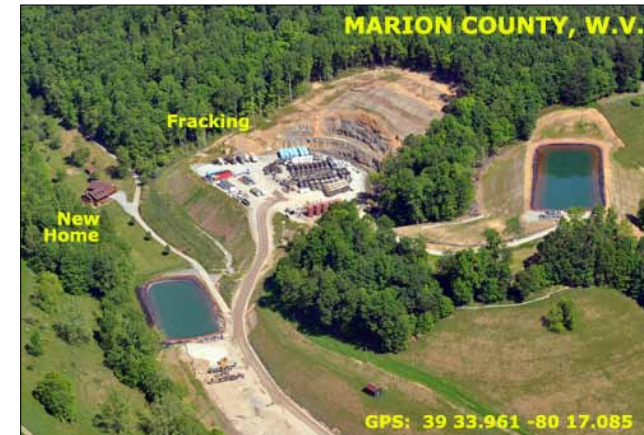
Keeping operations like these out of flood plains is a smart idea. Photo courtesy wvhostfarms.org and Bob Donnan.
