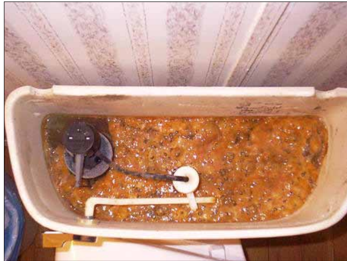
Um, hello, DEP? Contaminated well water created this disgusting brew in a Prenter resident's toilet tank. Photo by SSP
