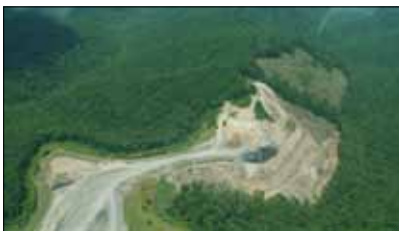
The MTR mine beside KSF. Though approximately one-fourth of the permit (100 acres of the total 413 acres) was mined between 2014 and 2015, the additional 300 acres has not been disturbed and will not be mined! Flyover courtesy SouthWings.org
