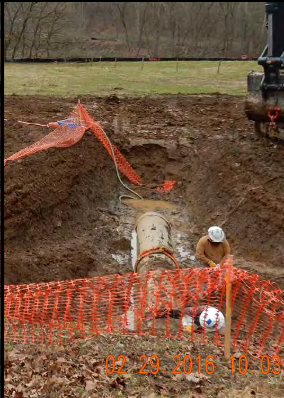
Receiving pipe pit before and after the pipe was bored under the roadway
