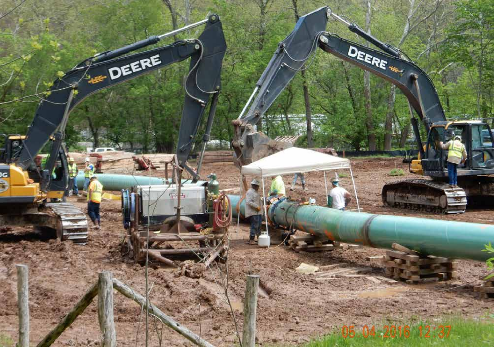
The pipeline section to be buried under the stream bed is being fabricated here.
