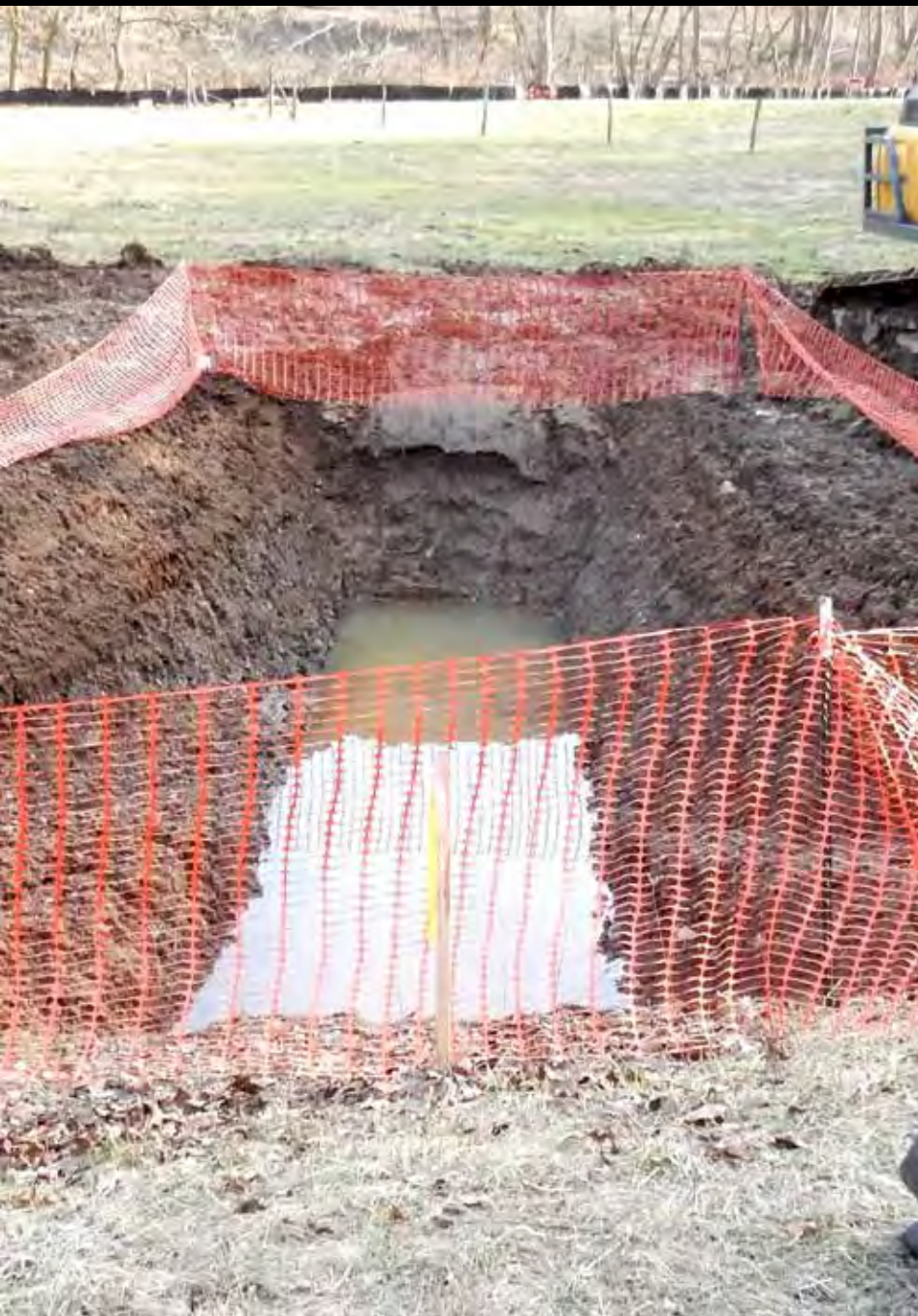
Receiving pipe pit before and after the pipe was bored under the roadway
