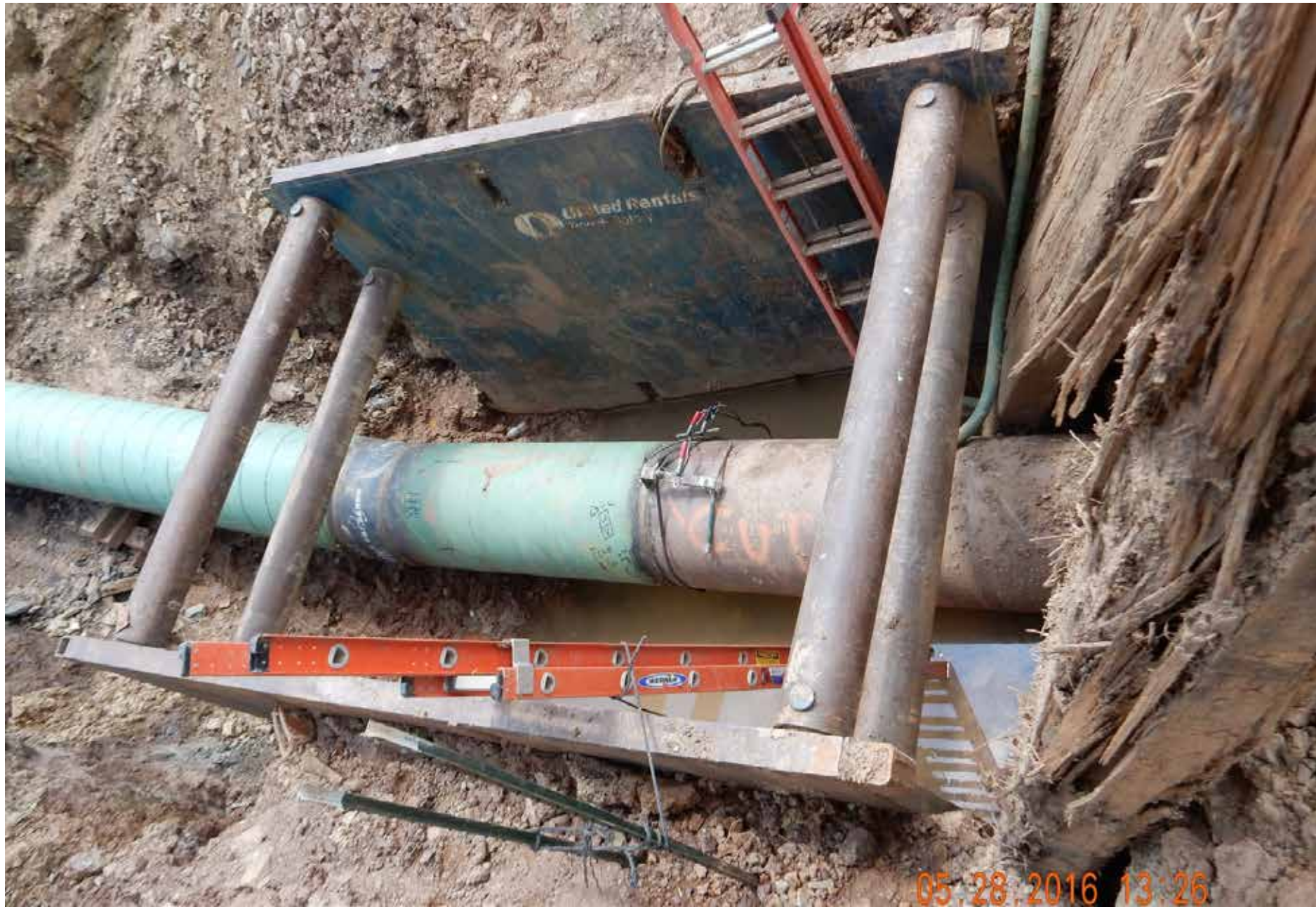
Exit end of the pipe after going under the road
