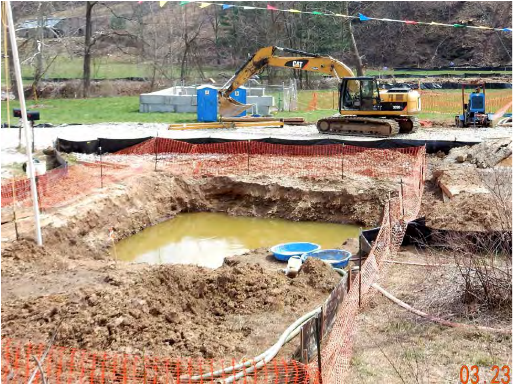
Example of a receiving pit filled up with water
