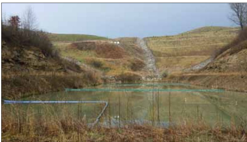
A "reclaimed" valley fill at an MTR site, still a source of pollution entering local waterways.
