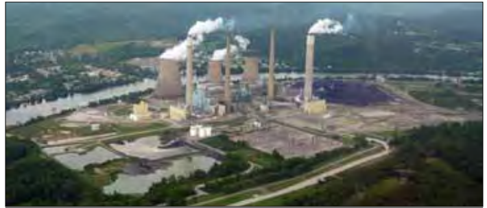
While serving as an aerial guide for WV filming for Time to Choose, Vivian snapped this shot of AEP's John Amos power plant near Charleston, WV.
