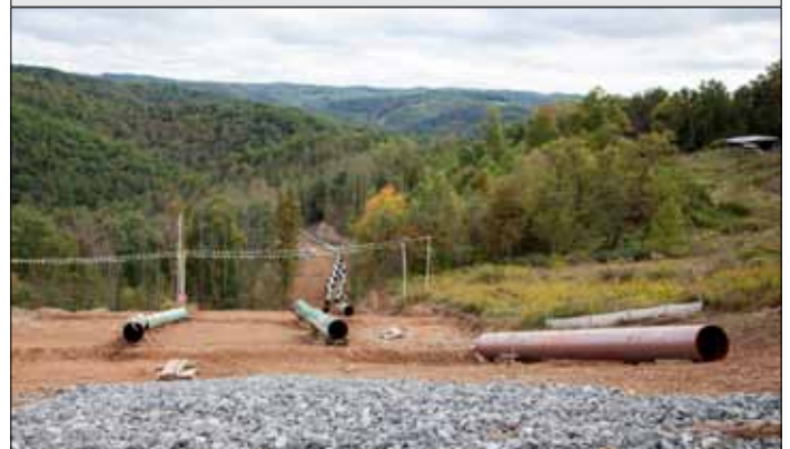
Construction of part of the Stonewall Gas Gathering Pipeline is underway in Lewis County, WV. This stretch of pipeline has a "mere" 36-inch diameter. Photos by Keely Kernan, keelykernan.com .
