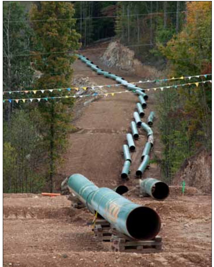
Construction of part of the Stonewall Gas Gathering Pipeline is underway in Lewis County, WV. This stretch of pipeline has a "mere" 36-inch diameter. Photos by Keely Kernan, keelykernan.com .
