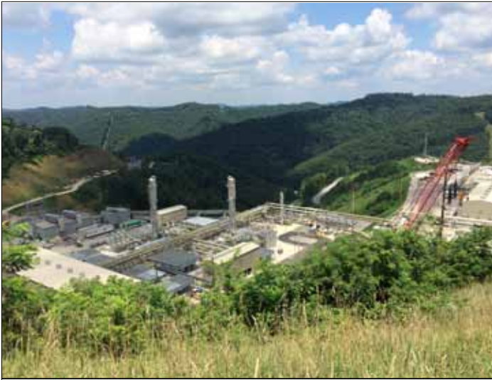
Part of the MarkWest gas processing plant in Mobley, Wetzel County, one of several such scenes OVEC board members pondered on their tour of Fracklandia. Photo by Janet Keating.
