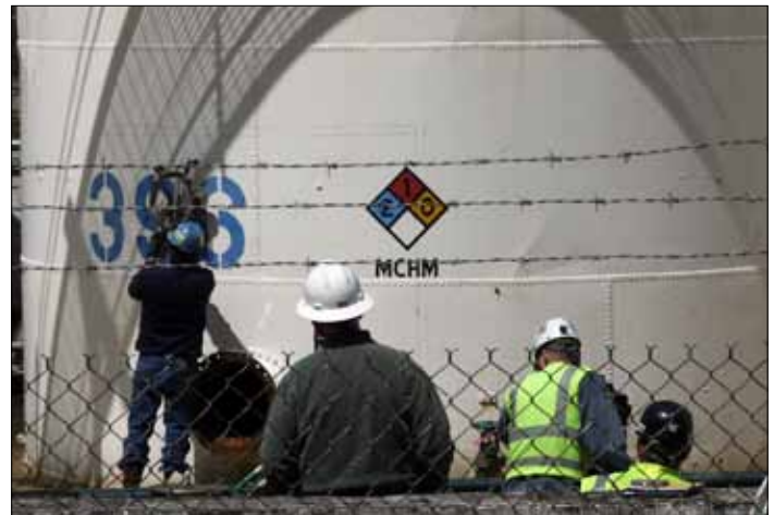
In April 2014, officials began opening tank 396 at Freedom Industries. The tanks are now gone, but the worries are not.
