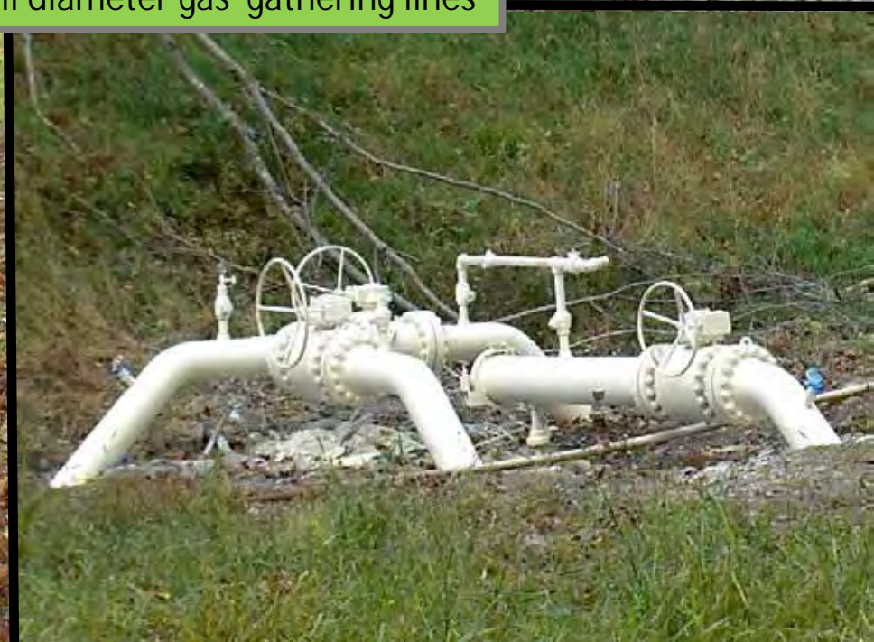
Assorted valve groups on small diameter gas gathering lines
