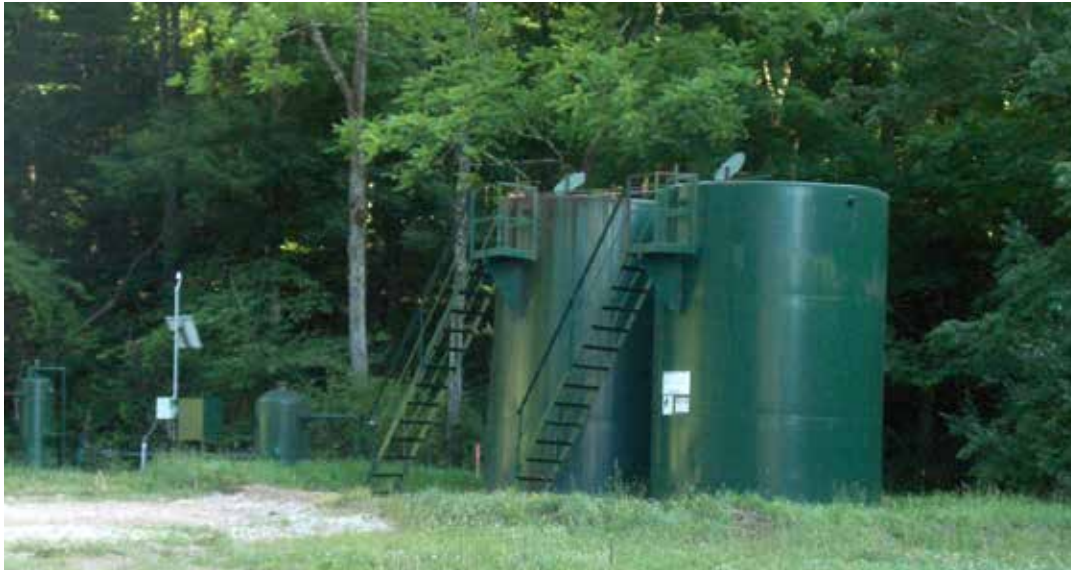
Condensate and Brine Storage Tanks on Well Pads
