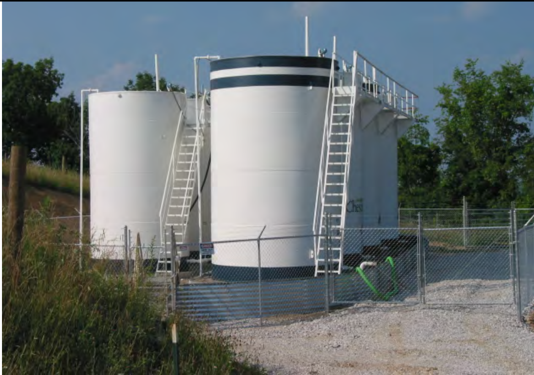
Condensate and Brine Storage Tanks on Well Pads
