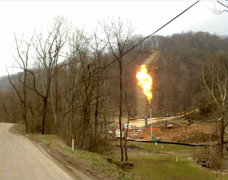
New Dominion gas plant along the Ohio River in SW Marshall Co. WV
