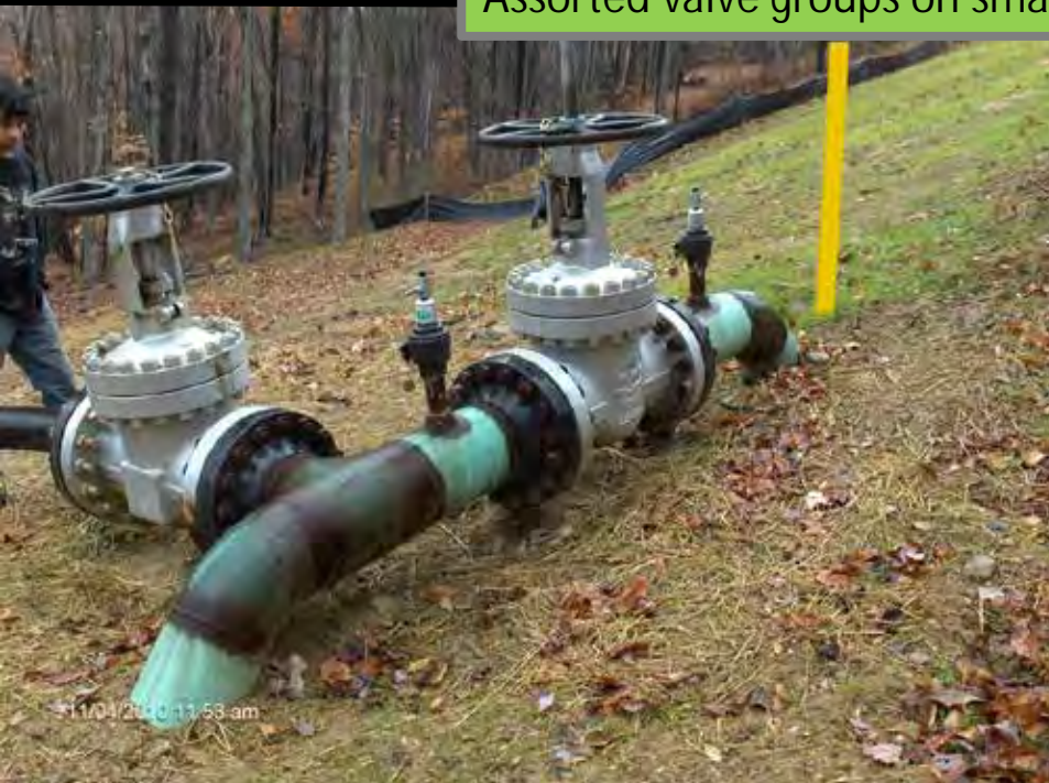
Assorted valve groups on small diameter gas gathering lines
