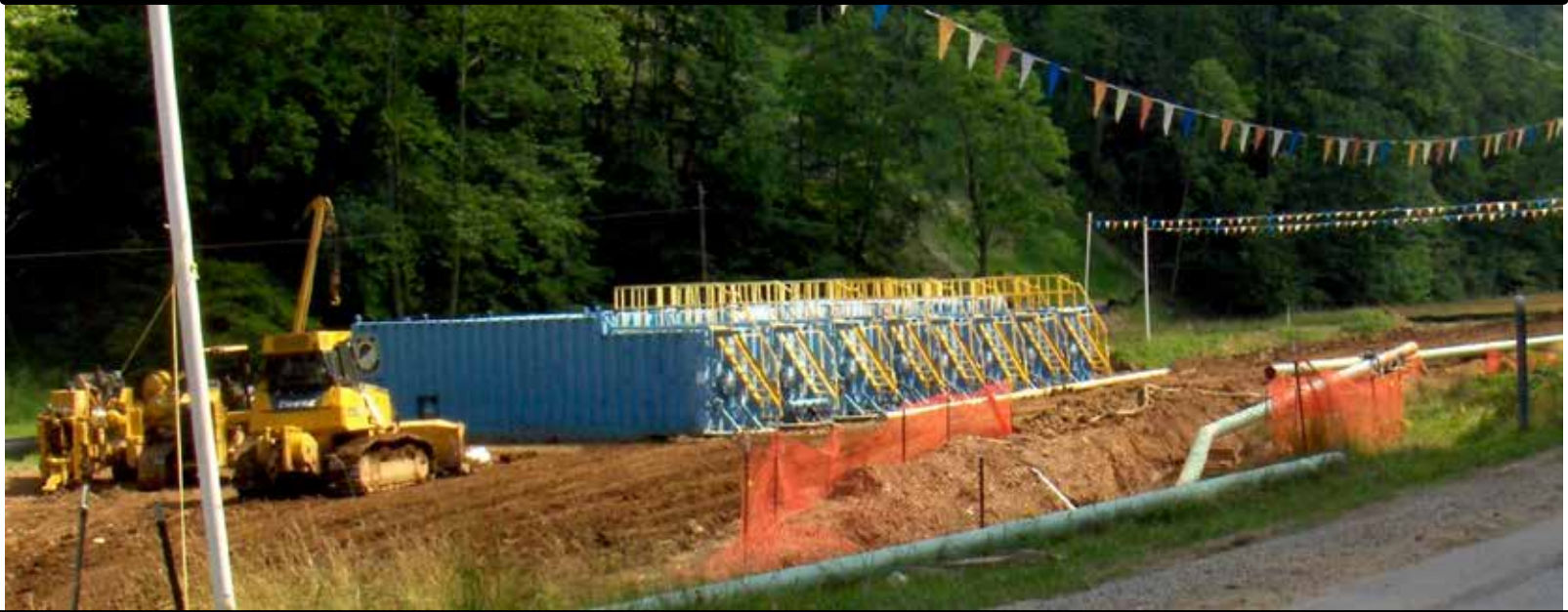
Temporary Fresh Water Storage for pipeline pressure test
