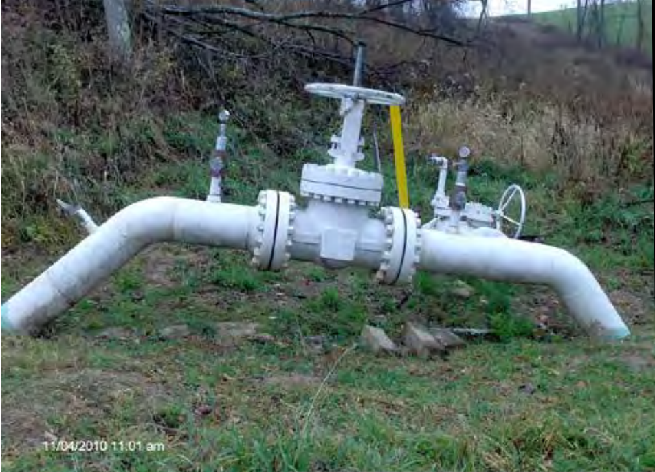
Assorted valve groups on small diameter gas gathering lines
