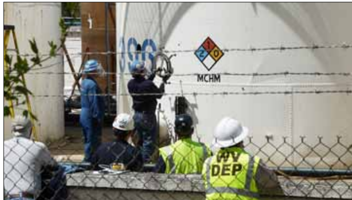
On April 24 the U.S. Chemical Safety Board began cutting open a MCHM tank at Freedom Industries, so that inspectors could enter the tank. The activity stirred up the sickening licorice-scent once again.
