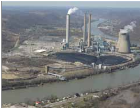
Outdated coal-fired power plants are major polluters.
