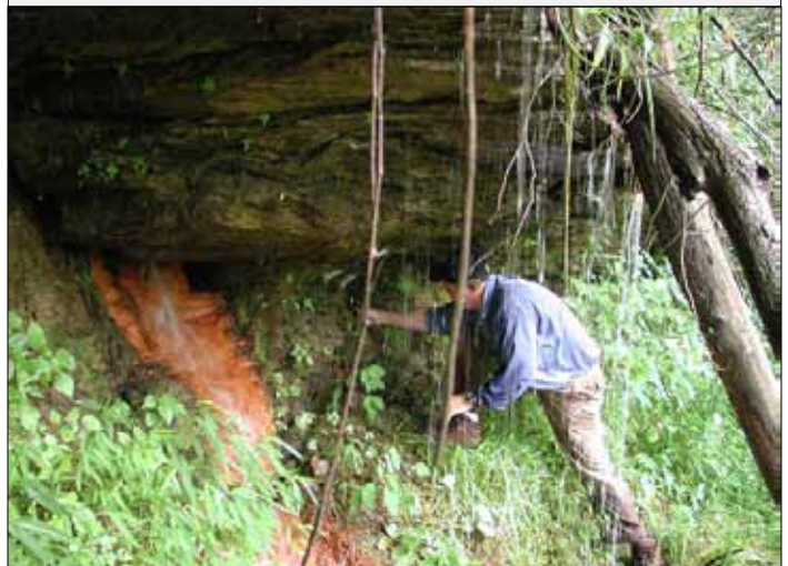
Dangerous situation? Polluted water pours out of a rock outcropping just downstream of a coal sludge dam in Mingo County. The rock is said to stretch back under the impoundment.
