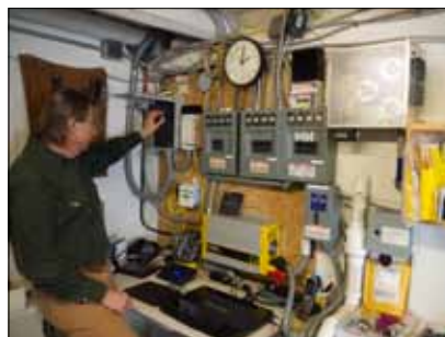
Janowski at the automated control panel for his off-grid power system. Photo by Vivian Stockman. Top two photos by Mickey Janowski.
