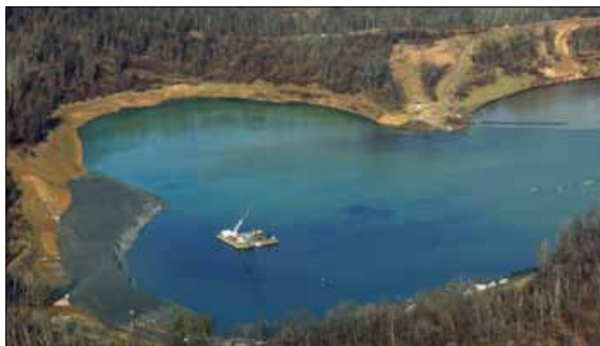
Above: At left, note the failed area of the embankment at CONSOL's Harrison County, W.Va. coal sludge dam. Below: Dwellings near the sludge impoundment. Flyover courtesy SouthWings.org.
