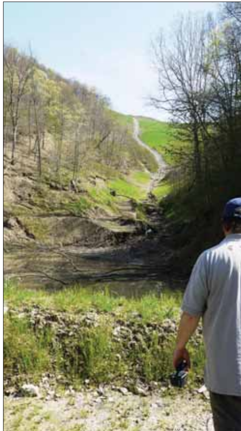
A valley fill from below. This is not “sustainable use” in any way, shape or form.
