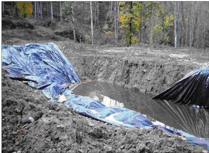
Just in case anyone doubts the need for comprehensive drilling regulations AND constant oversight, this is a waste pit at a Waco (Ike Morris) operation in Doddridge County. Note the care taken with the liner.
