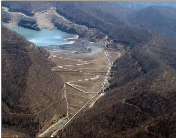
The Brushy Fork coal impoundment in Raleigh County, WV, which will, when completed, hold more than 8 BILLION gallons of coal sludge and be 900 feet high.
